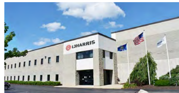
Londonderry, New Hampshire, U.S.A. facilities
